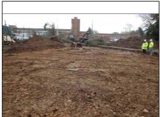
Stripped Watching Brief area, facing south
