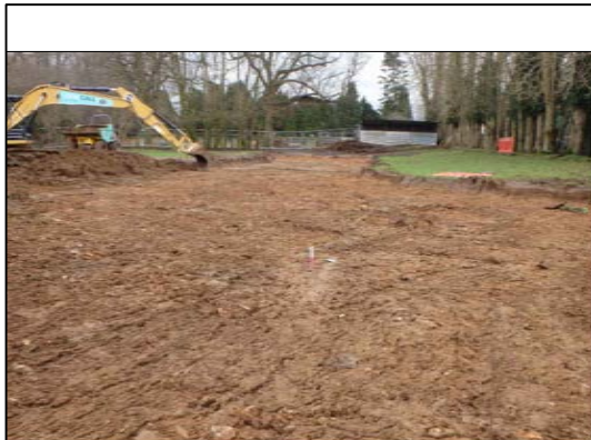
Stripped Watching Brief area, facing east
