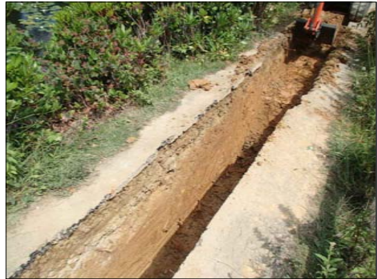
Moat repair trench
