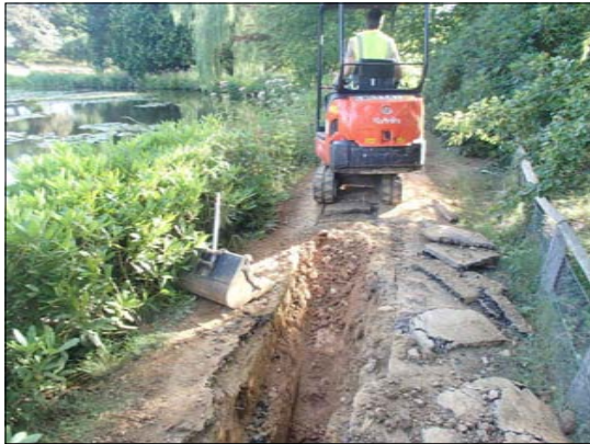
Moat repair trench
