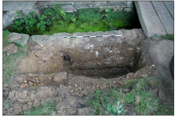
Sluice repair channel section
