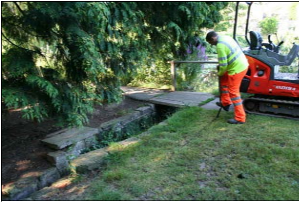
Excavation of sluice repair channel
