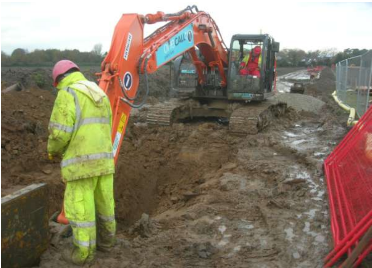
Plate 4. Phase 1. Topsoil strip. Plate 5 (below) Phase 2. Cutting trench for pipe
