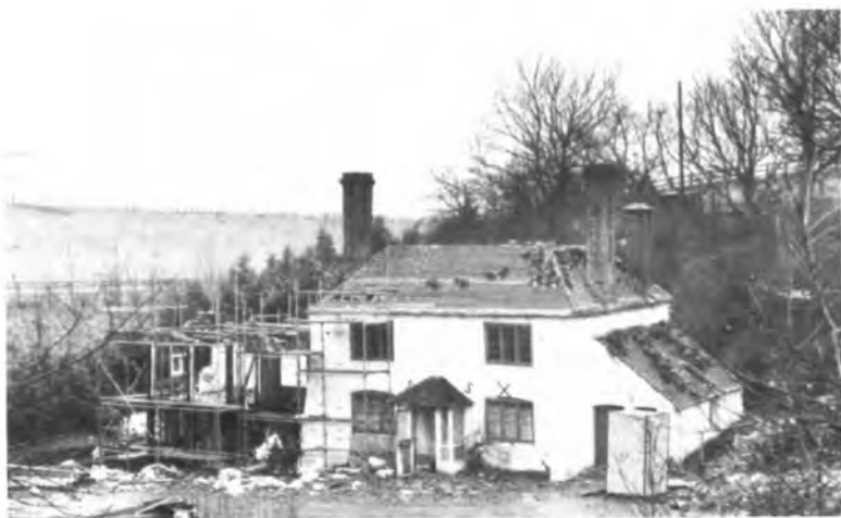
Mill House during demolition. Looking south-west.
