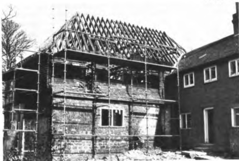
Stone Farm being dismantled. Looking north-east.
