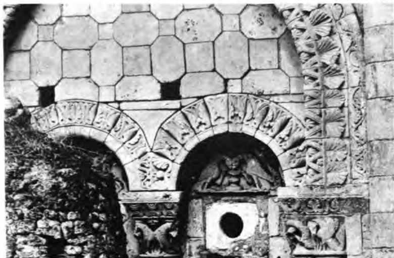
Villesalem, Priory Church, west Façade, Detail of Arcading (Photo: Courtesy G. Zarnecki and Courtauld Institute of Art, London).
