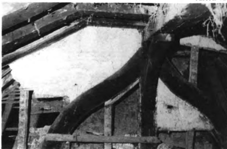
(Photo: M.G. Heenan) Horton Manor: West End of Hall Roof.
