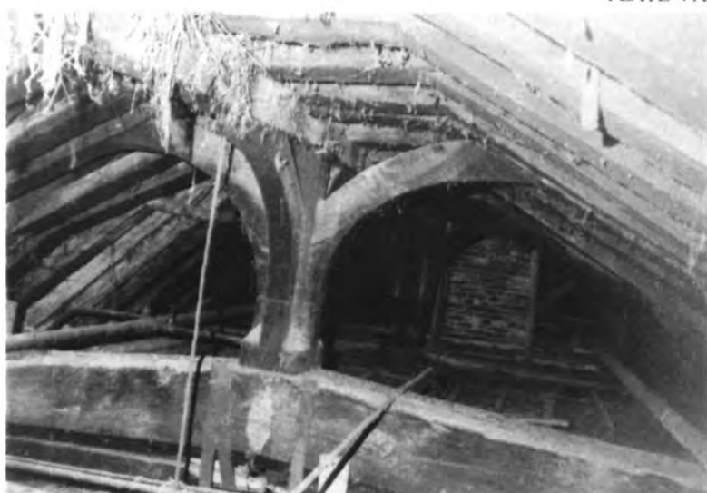
(Photo: M.G. Heenan) Horton Manor: Hall Roof looking South.
