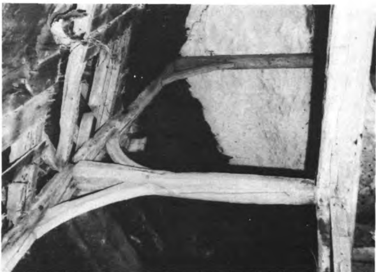
Horton Manor Chapel: Nave Roof, looking North-east with Chancel Area below.
