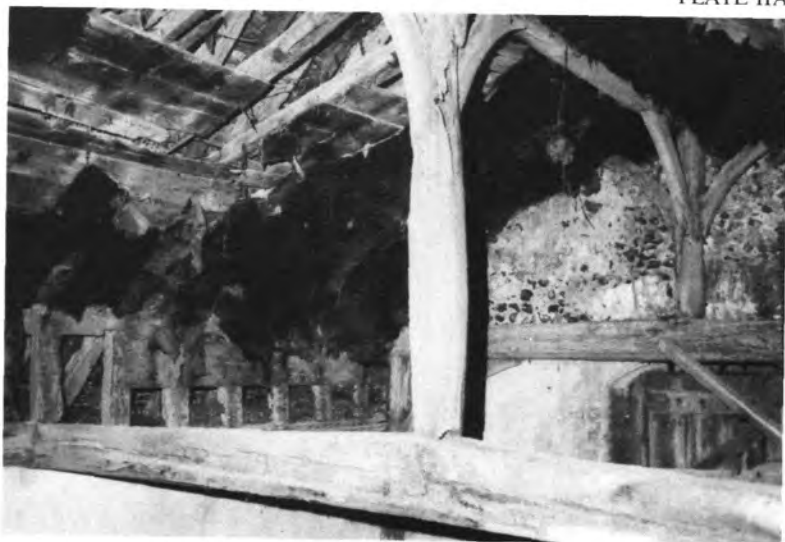
Horton Manor Chapel: Nave Roof, looking South-west.
