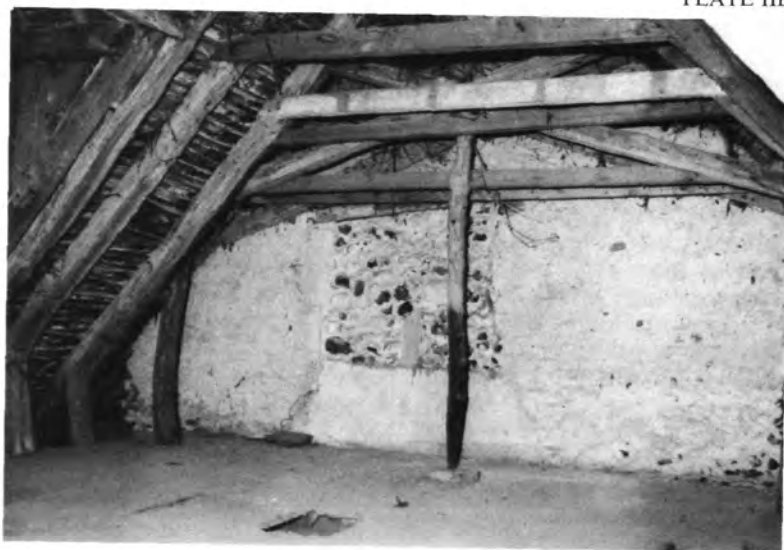
Horton Manor Chapel: Chancel Roof, looking South-west.
