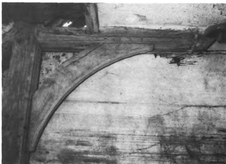
Horton Manor Chapel: Northern Half of western Truss in the Nave Roof.
