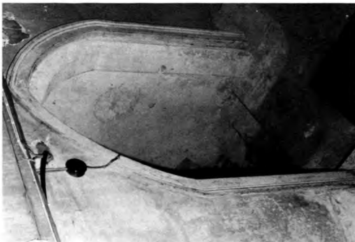
The Basement Doorway to the Tower, Stone Castle, looking South-east.
