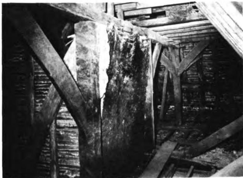
The Roof looking East, showing Smoke-bay Partition and Crown Post.
