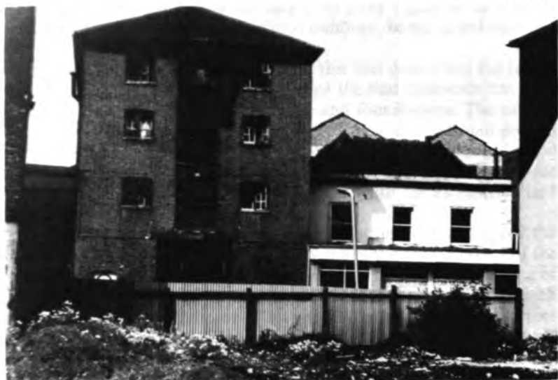
Westborough House, east Elevation.
