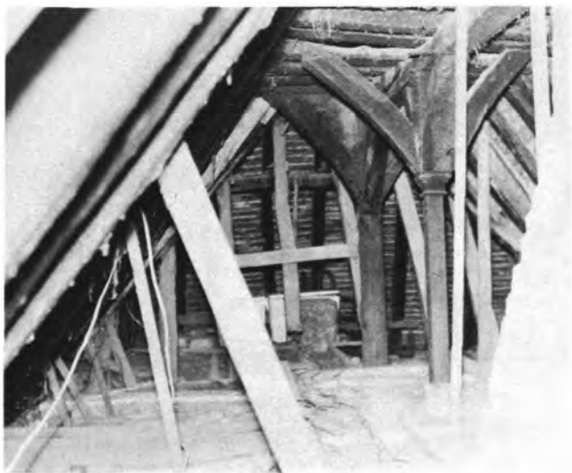
Plate IB. Inside the north End of the Roof.
