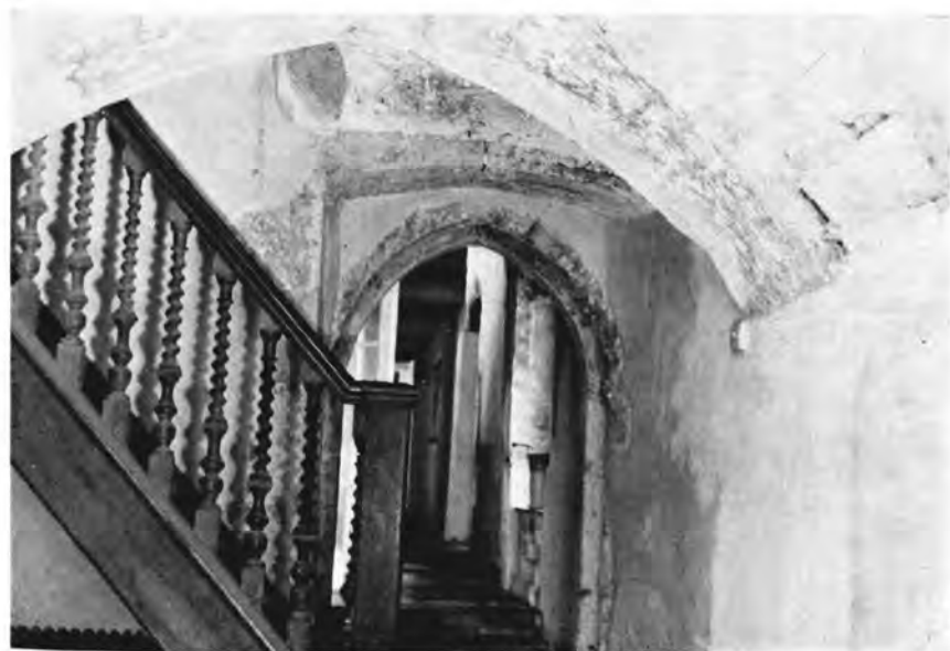
B. Inside Vault under Chaplain's Room.
