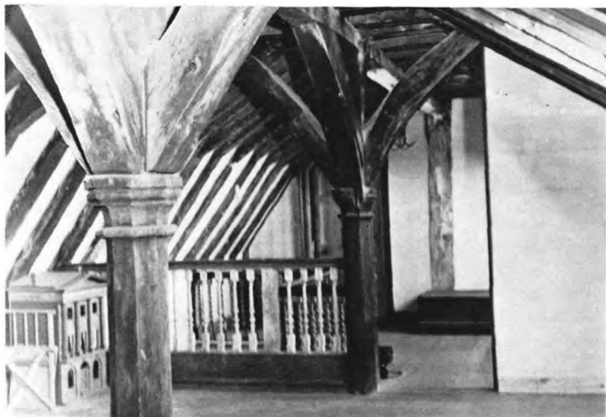
A. The Crown-post Roof.
