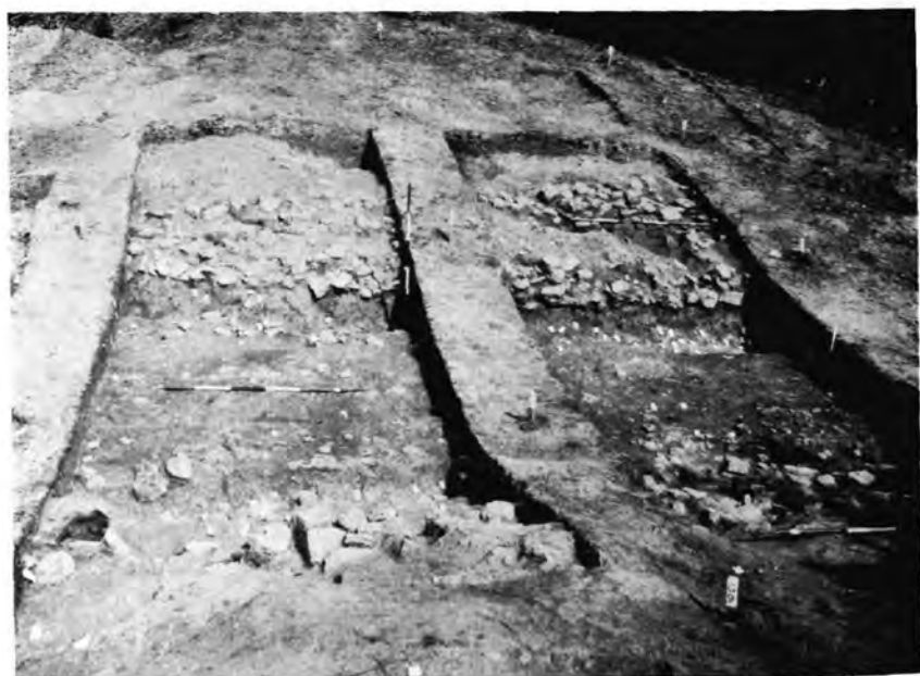
East Entrance of Fort I, looking South. General View of outer Entrance, showing revetted Rampart-ends, Gullies and Roadway. The vertical ranging rod stands in the southern gully; the horizontal rod, along the middle of the roadway.
