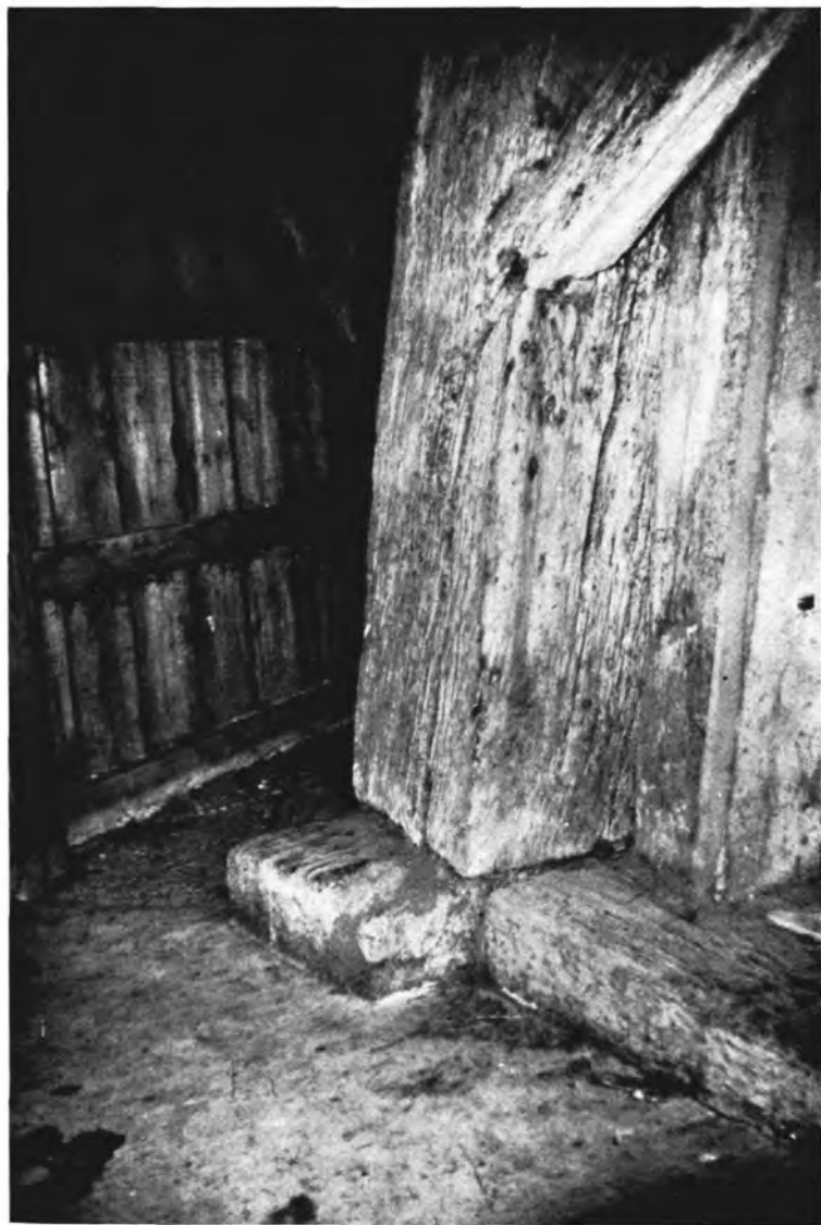
Brookland Belfry. Foot of the north-west Post, showing notched-lap Joint, at the lower end of a diagonal Brace.
