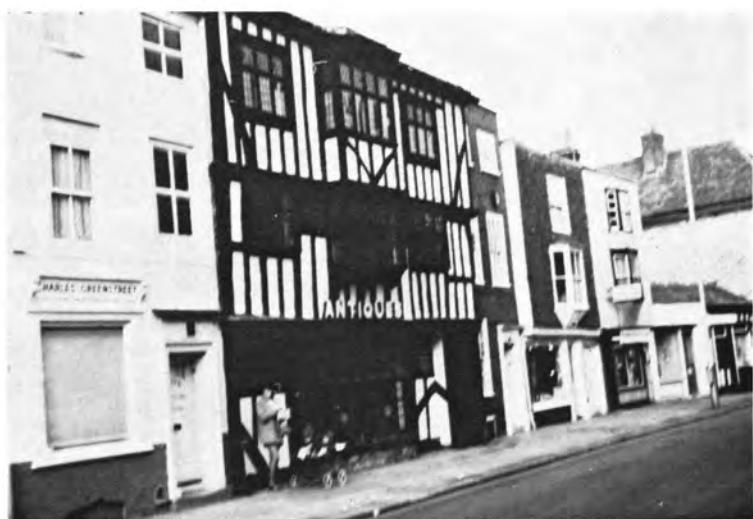
A. The Street Front of no. 17 Palace Street.
