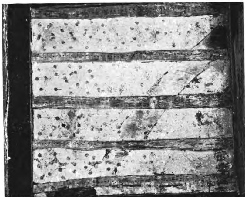
B. Decoration on lime-washed Daub Filling between Studs in lower half of Partition shown in Plate 1B.
