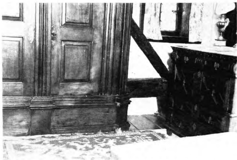
B. Remains of 1495 Roof Timbers, and the 1740 Wardrobe built around them.
