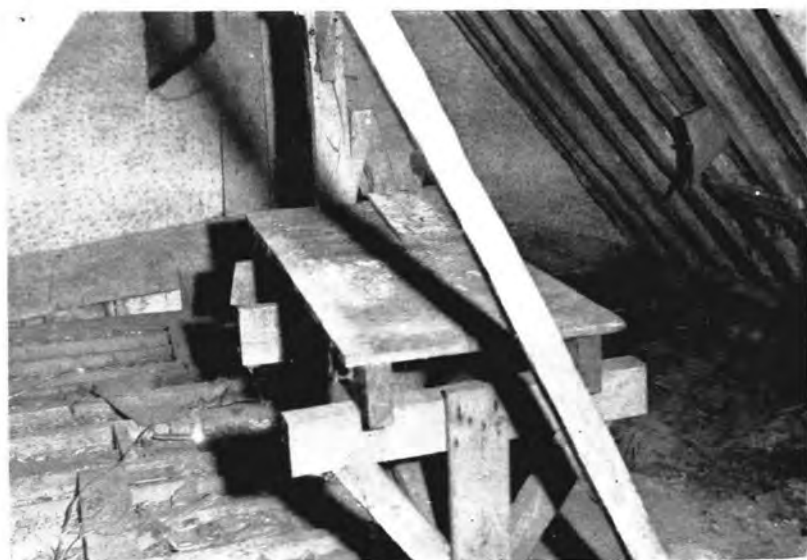
B. The roof of the smaller wing.
