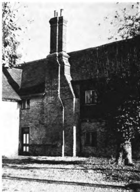
A. The seventeenth-century chimney breast.
