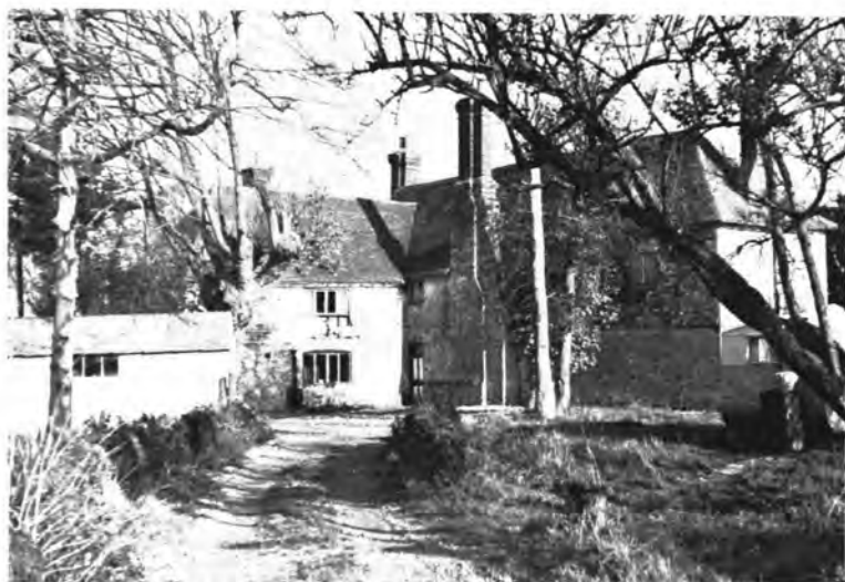
A. Harringe Court, view from the south-west.
