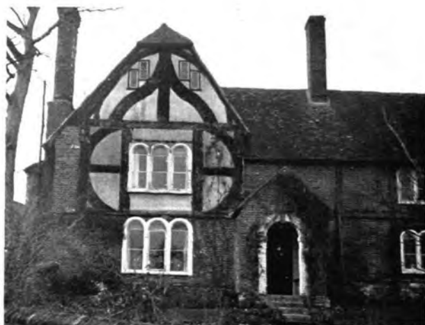
B. Rooting, Exterior from E.
