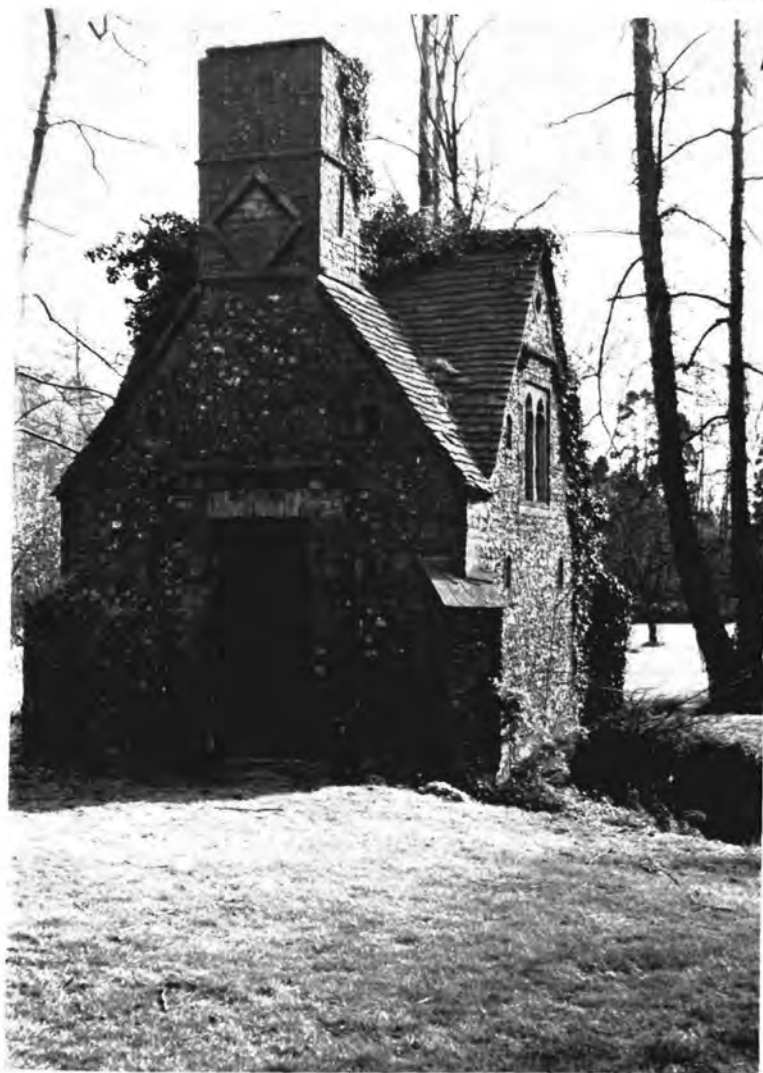
The Vale Maschal bath house, showing small blocked windows of rubbed brick.
