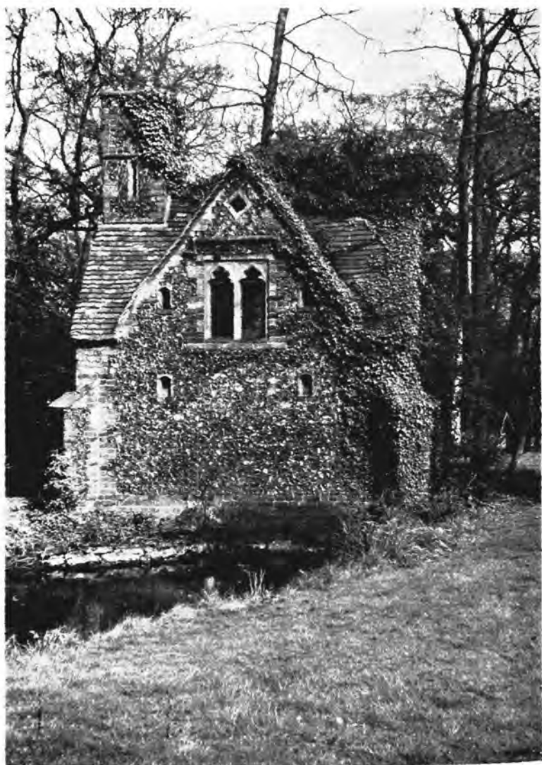
The Vale Maschal bath house, showing Gothic-style glazed windows.
