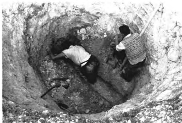
B. View of the Shaft. Removing the filling below Level 7.
