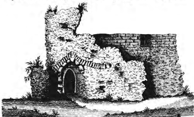
Fig. 3. South View of the Remains of Higham Abby; p. 122.
