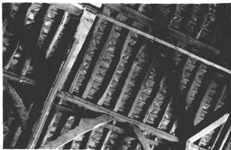
B. Austin Lodge, Eynsford: Halved Scarf and eccentric Braces.
