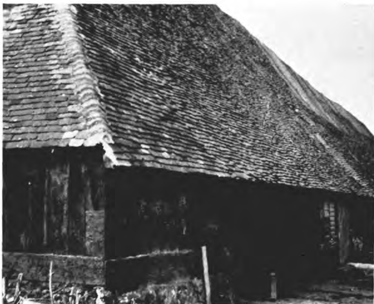
A. Frindsbury: S.E. Corner, showing Cladding.
