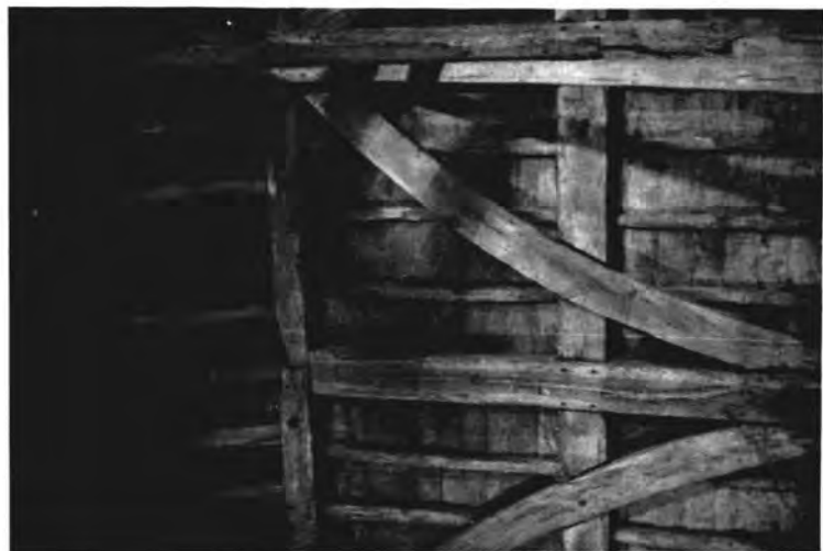
B. Nettlestead: Braces in Wall-frame.
