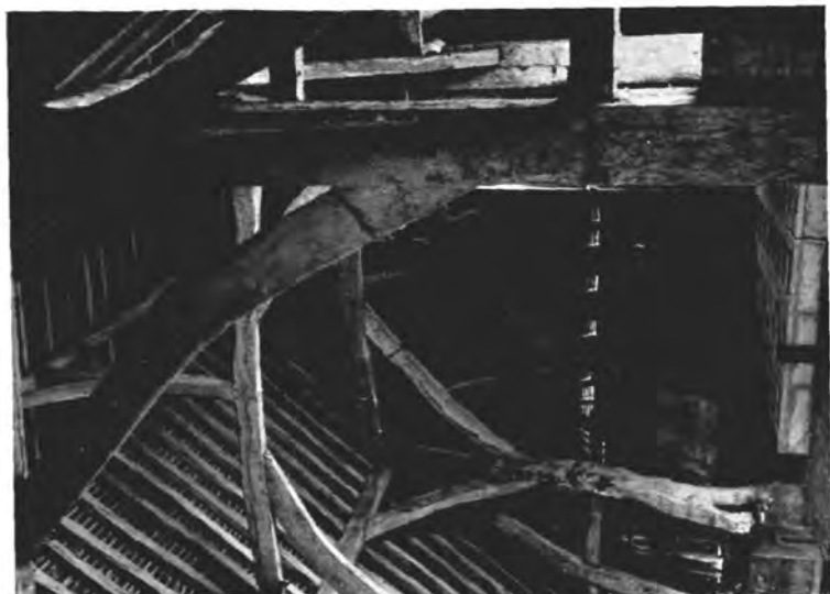
S.E.R. B. Faversham Minor: S.W. part, showing unshaped Posts.
