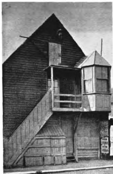
A. Building at the Horsebridge, Whitstable now demolished. Nightly orders to the dredgermen were issued from the oriel window.
