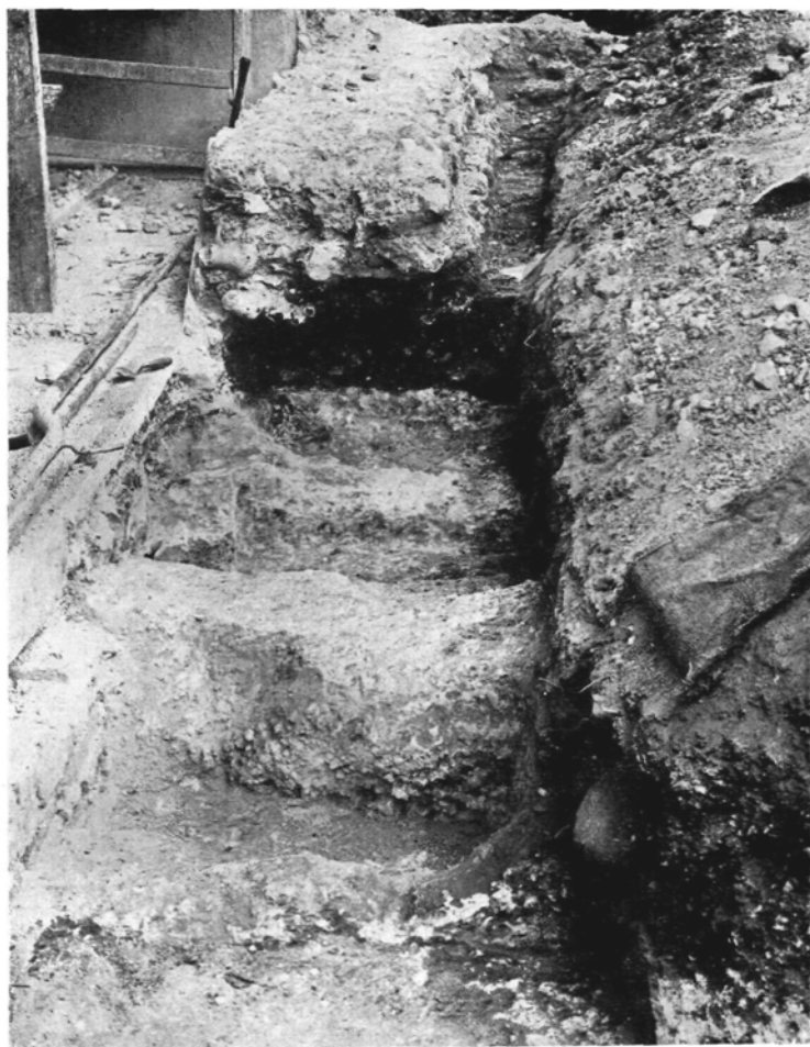
KESTON CHURCH, KENT. East wall rebuilding, 1950.
