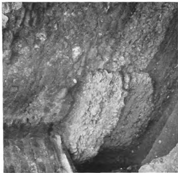
PLATE I (2). BURGATE STREET SITE. Clasp buttress at north-west corner of building.
