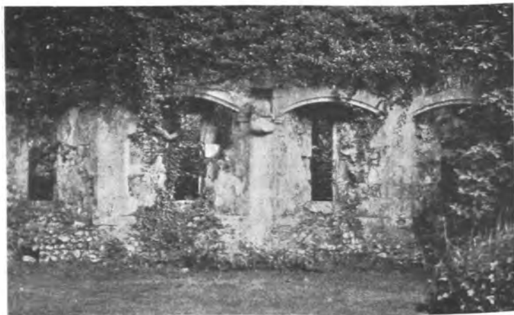
WINDOWS IN WEST WALL OF FORENSIC PARLOUR.
