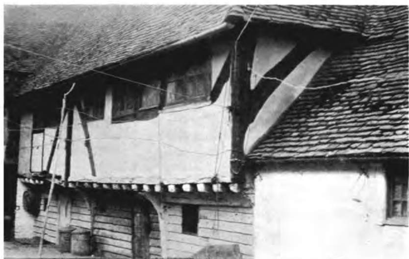
Detail at the back of the Hall.
