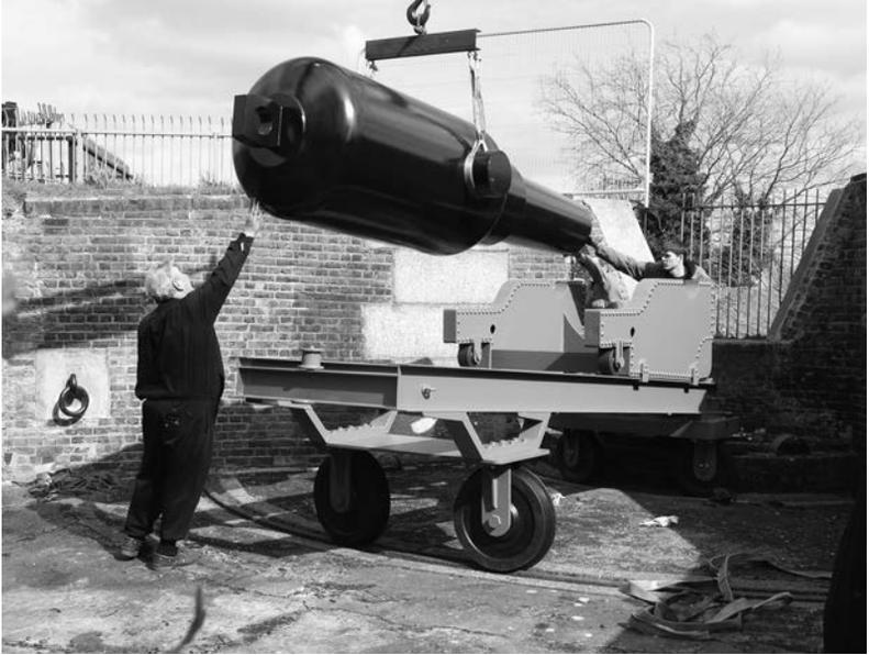
Fig. 4 Mounting of a replica 9-in. RML in the Garden Face, with backing blocks for an intended iron shield in the background (Victor Smith 2010).
