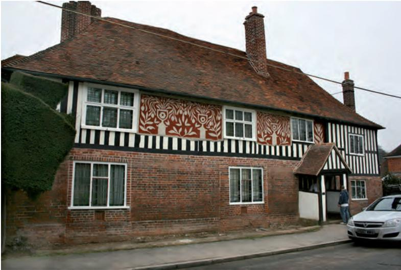
View of south elevation of main range of house, showing close studding and painted plaster
