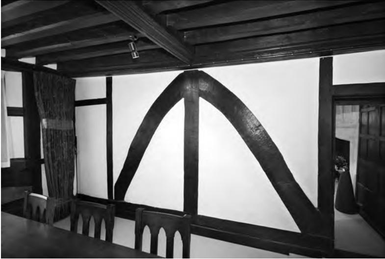
West wall of hall, showing framing of earlier medieval open-hall (note moulded beams and chamfered joists overhead)
