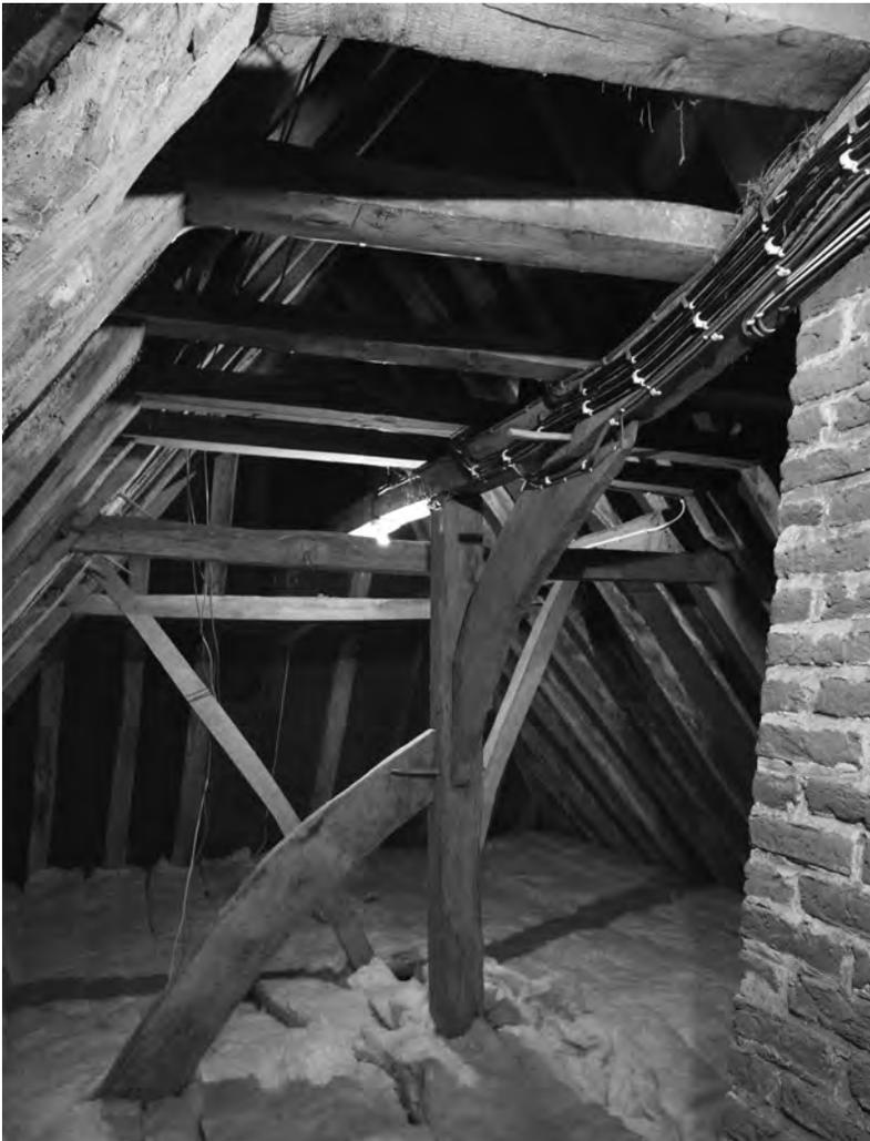
View of attic, looking east, showing crown-post (note single down brace)
