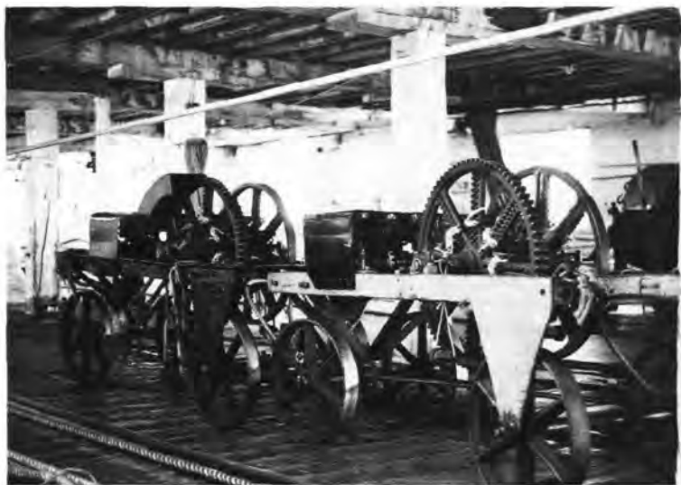
Two of the original Chatham ropery jack wheels that were delivered to the yard in 1811 having been constructed by the Henry Maudslay Company
