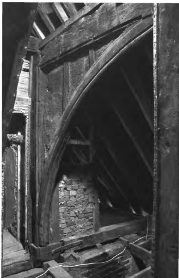
East arcade-brace (south bay, looking north) showing planking rebate
