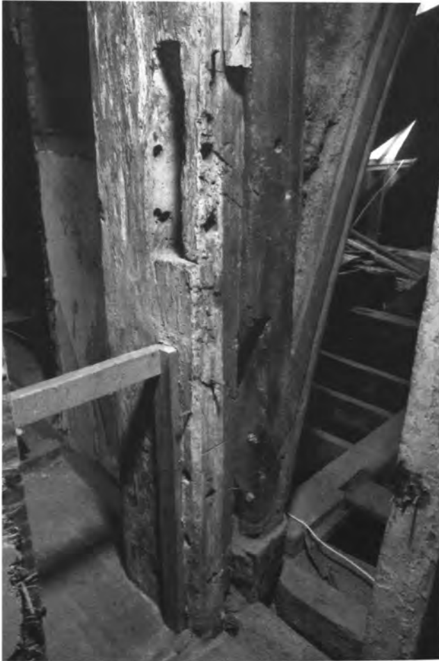
North end truss arcade-post, looking south-east
