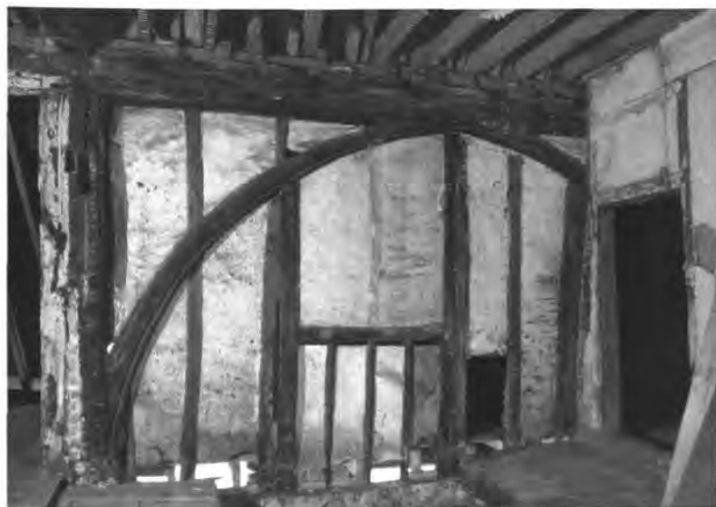
East arcade (south bay, looking west) showing arcade-braces and inserted window
