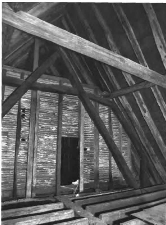
Central roof truss, looking north showing passing braces
