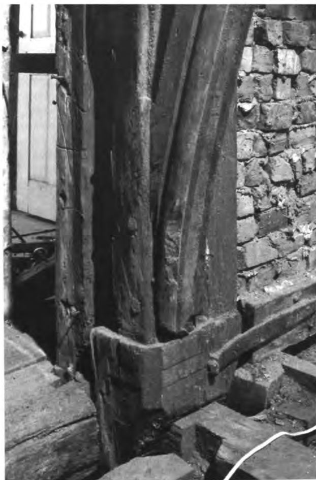
Central truss arcade post, looking north-east
