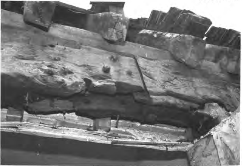
Face-splayed and tabled scarf (east arcade, south bay)
