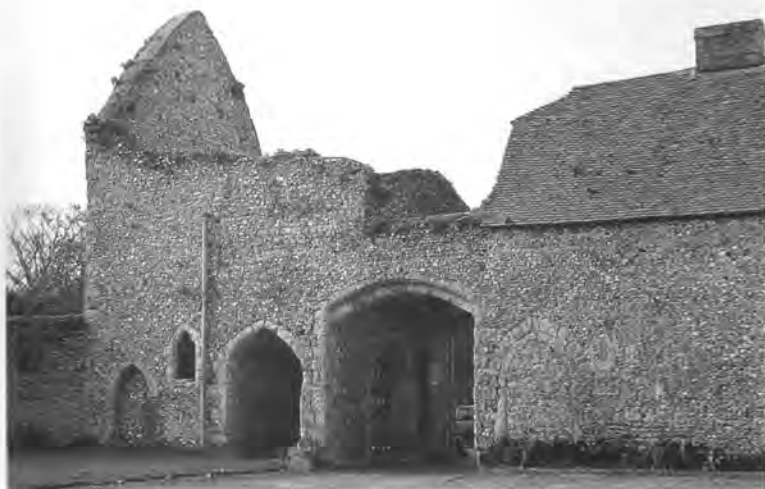
North façade of the gateway and adjoining area. The eastern blocked doorway formerly opened into a small ground-floor room, the western one probably led to a stair to the first floor. The area above and to the east of the gate formed a large, well-appointed chamber. Photo: the author.
