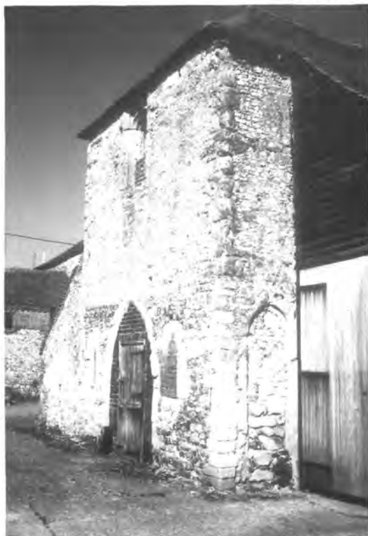
Porch of the Great Hall, showing the original entrance and the small blocked doorway to the intra-mural stair. Photo: the author.
