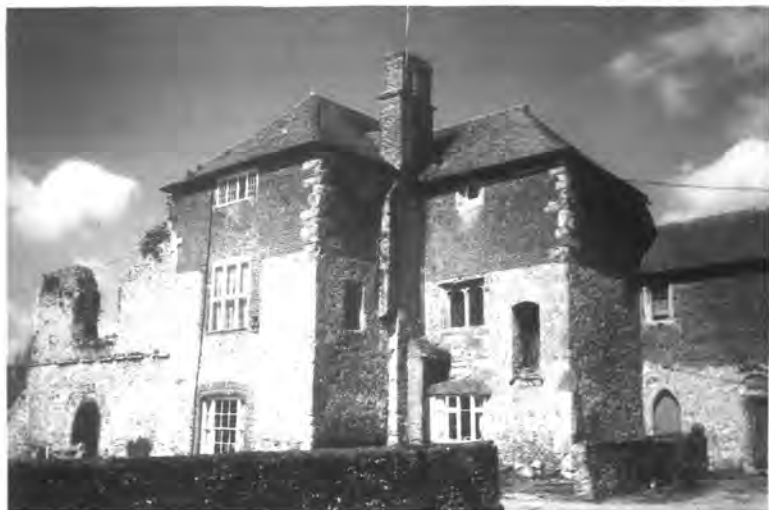
The private accommodation from the south-east. To the left is the ruined chamber range of the late thirteenth century. The central ranges were built in stone in the late fourteenth century and heightened in brick in the late fifteenth. The passage linking the private apartments to the hall can be seen to the right. Photo: the author
