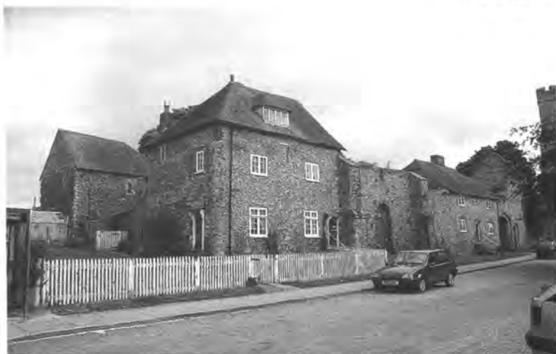
Gatehouse range from the south-west showing the two former garderobe blocks projecting from the west lodging range. Photo: the author.
