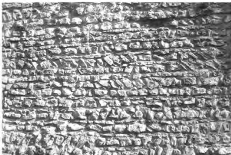
St Leonard's Tower: typical coursed ragstone walling (south face).
