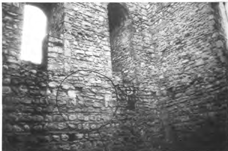
St Leonard's Tower: window seat and tufa brackets (circled).
