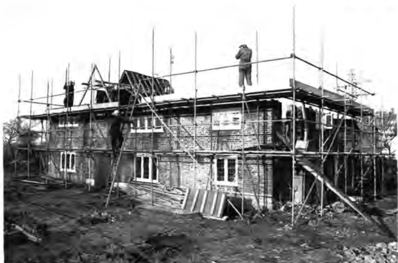
Longport House, Cheriton, during dismantling. Looking north-west.
