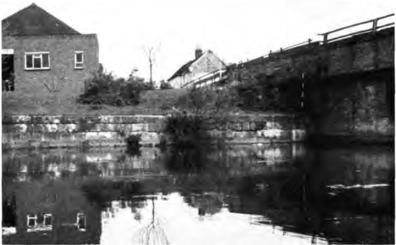
Hythe, Duke's Head Bridge. Looking east. Scale: 2 m.
