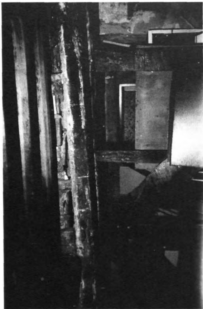
The Hall Ceiling after the Removal of the Plaster.
