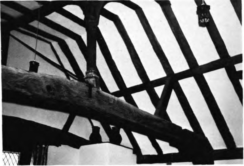
The Crown-Post Roof of the Old Canonry.
