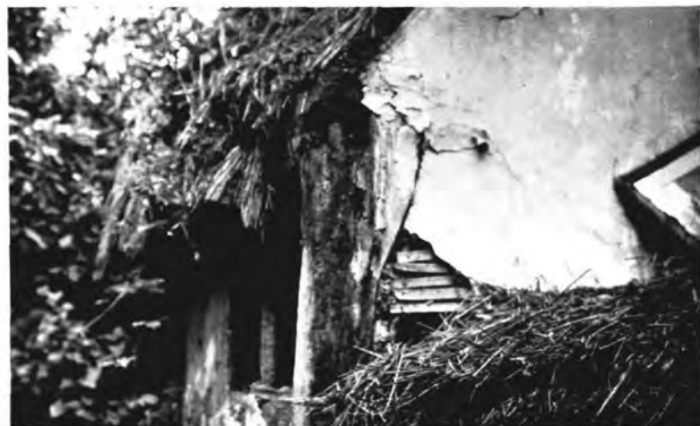
B. Post on West Side.
