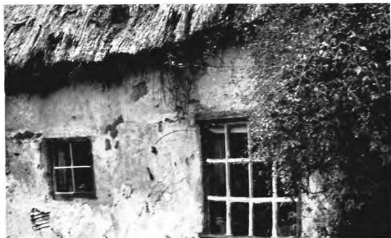
A. Windows on East Side.
