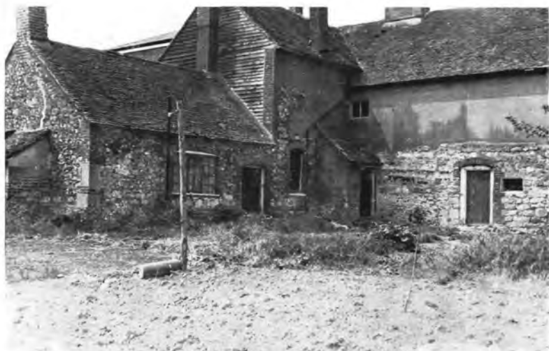
A. General view of cottages on east side showing the N-S wall on right and E-W part with outbuildings on left.
