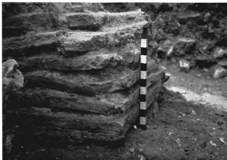
Brick jamb at entrance to hypocaust. ROMAN VILLA IN COBHAM PARK.
