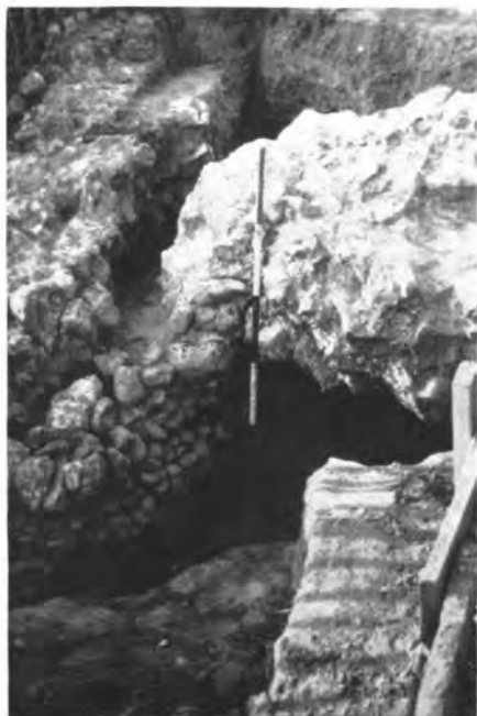
S.W. corner of fort. Joint (behind pole) of buttress and wall (falling away to left)
