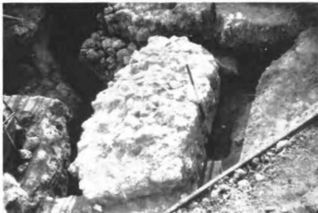
S.W. corner of fort. Surviving portion of Internal buttress (fort wall above)
