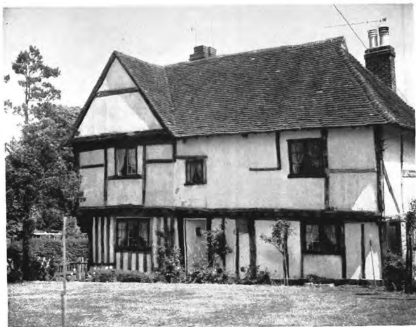
The original farm house of Boarley Farm, Boxley
