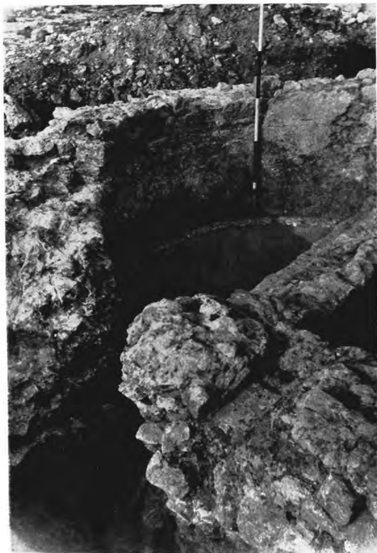
The apsidal bath of the frigidarium , showing (left, below) the period 2 drain of the bath and (above, in the foreground) the original drain of the frigidarium floor.
