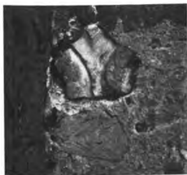
(b) Bifurcation of arcading and a fragment of tooled Caen-stone re-used in E. face of NW. buttress of tower.
