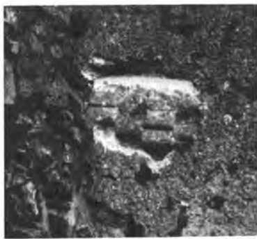
(c) Fragment of billet moulding re-used in E. wall of N. transept.
