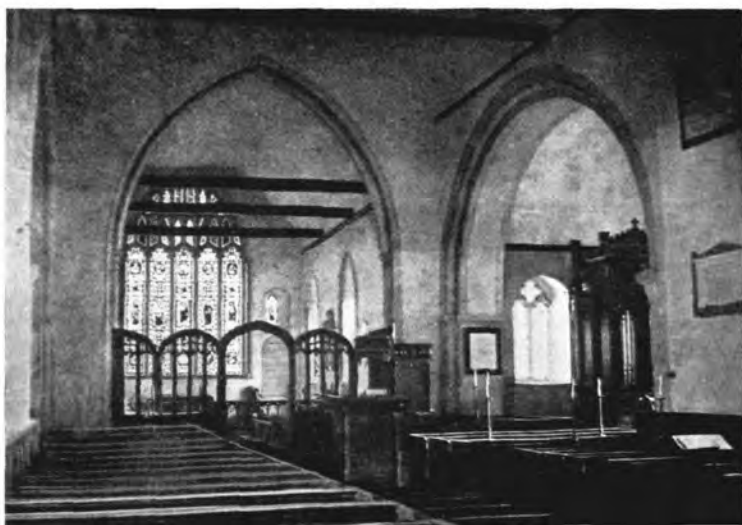
(b) Showing the rood-screen mutilated and the parclose gone, subsequently to 1857. From a photograph in the Vestry.
