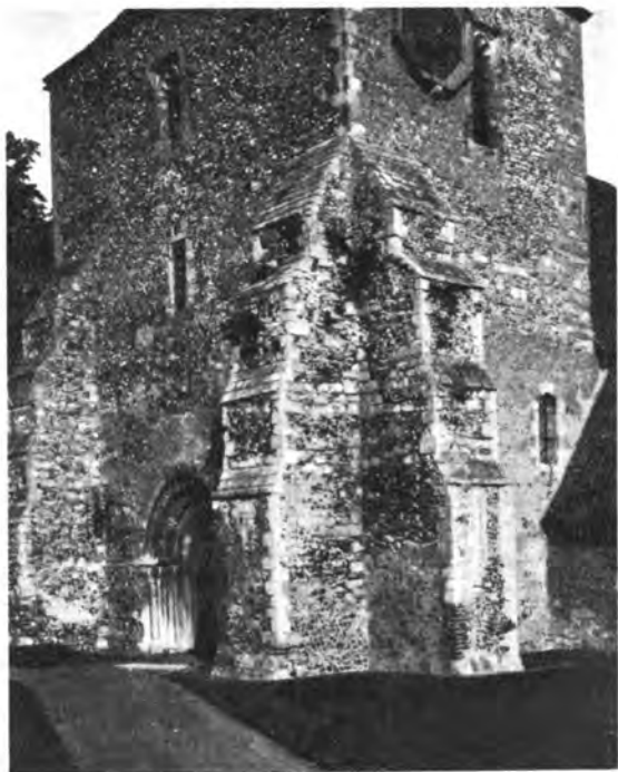
(a) West and South walls of tower showing re-used Caen stone.
