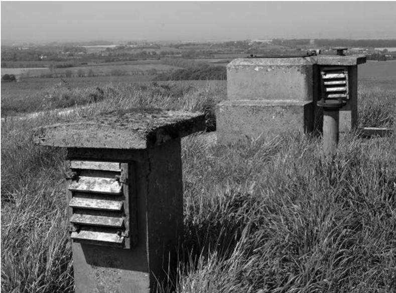
Fig. 9 Vent and entrance structure of the Clay Hill Royal Observer Corps underground post (Mark Harrison 2009).
