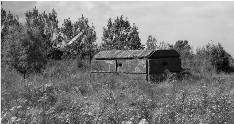
Fig. 5 Local variant pillbox on marshland overlooking the London-Margate railway. It had been painted green and given a timber facade to represent itself as the lambing shed marked on then current OS maps (Mark Harrison 2009).
